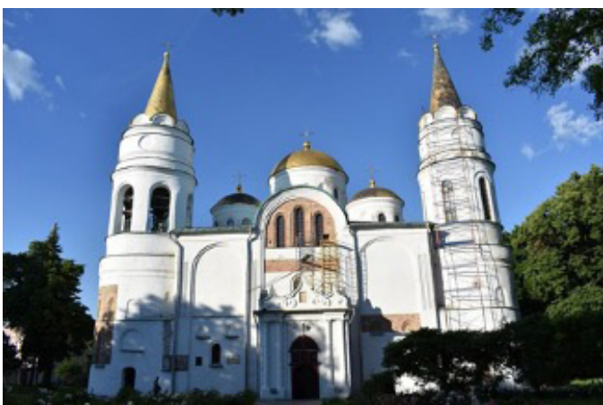
Savior Transfiguration Cathedral (1030s, with later renovations) in Chernihiv. View from the west with the damage visible on the southwest tower. Photograph by Anatolii Pobelian.
