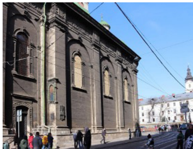
Dormition Church (1591–1629) in Lviv. View from the southwest with protective shields on windows. Photograph by Vasyl Petryk.
