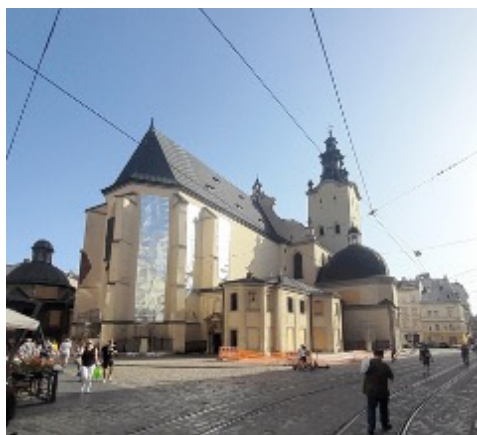
Latin Cathedral (begun in the 15th century) in Lviv. View from the northeast with protective shields on windows and metal fences around sculptures. Photograph by the author.
