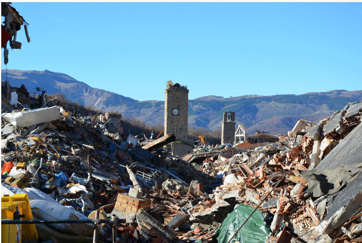
View of Amatrice buried under the rubble (November 2016) (photo: Francesco Gangemi)
